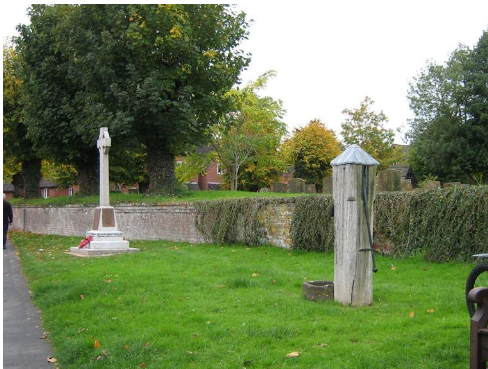
Listed War Memorial and non-designated Water Pump, Crown Street
